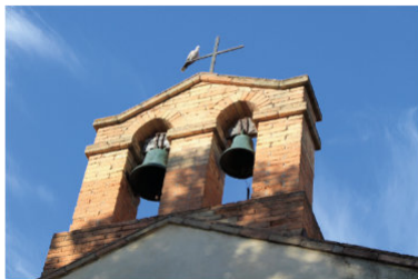
Detail of the bell tower
